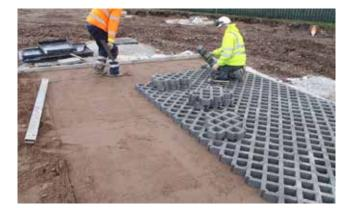
Several products were considered and dismissed before TERRAM's Truckpave was selected as the solution. Using Truckpave with a soil/seed/grass infill enabled large trucks to drive over the field to access the tank without damaging the grass. At all other times the area would look exactly like a normal school playing field and could be used by pupils.
