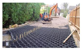
spread laterally reducing loads on the underlying soils. Without the cellular system, the surface would have become compacted and rutted with the forces pushing downwards damaging the tree roots and possibly killing the trees. Geocell was installed onto the level surface on top of a geotextile. The cells were filled with a type 1 road stone and compacted flat. A geotextile and binding layer were installed on top of the cells and the surface finished with small angular gravel.
