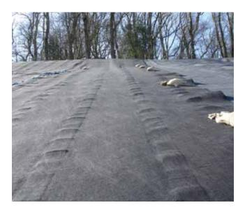
Later in the year, further product was supplied to the site: TERRAM RG4 as a capping geotextile for the northern flank restoration of cells 1 and 2 and TERRAM RG11 beneath a dual layer of a 6mm granite and 20/40mm granite at the base of cell 3A. Prior to supply of the Terram RG11 the product had passed an independent Environment Agency Cylinder Test to replicate the cells maximum 44m waste depth.
