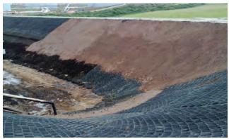
Geocell panels infilled with selected graded top soil.
