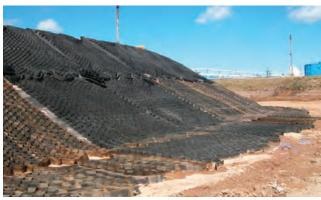
Geocell panels positioned and fixed prior to filling
