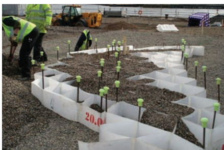
Terram Geocells, 220mm x 220mm, 3m x 6m panels, first layer
