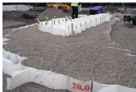
Terram Geocells, 220mm x 200mm, 3m x 6m panels, second layer
