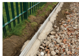
Edging kerbs installed
