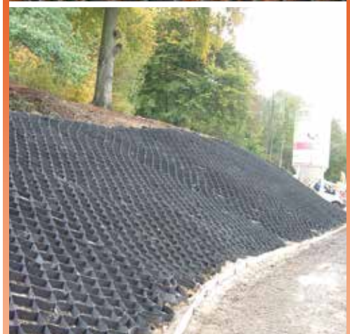
TERRAM GEOCELLS are anchored to slopes using U shaped - TERRAM Fixing Pins - these combined with the weight of the soil prevents slippage.
